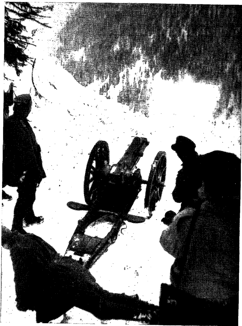
Figure 73.—75-mm mountain howitzer without shield.
