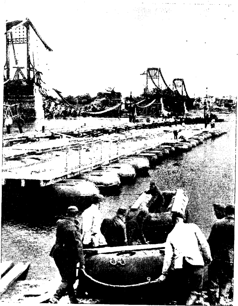
Figure 123.—Ponton bridge under construction.
